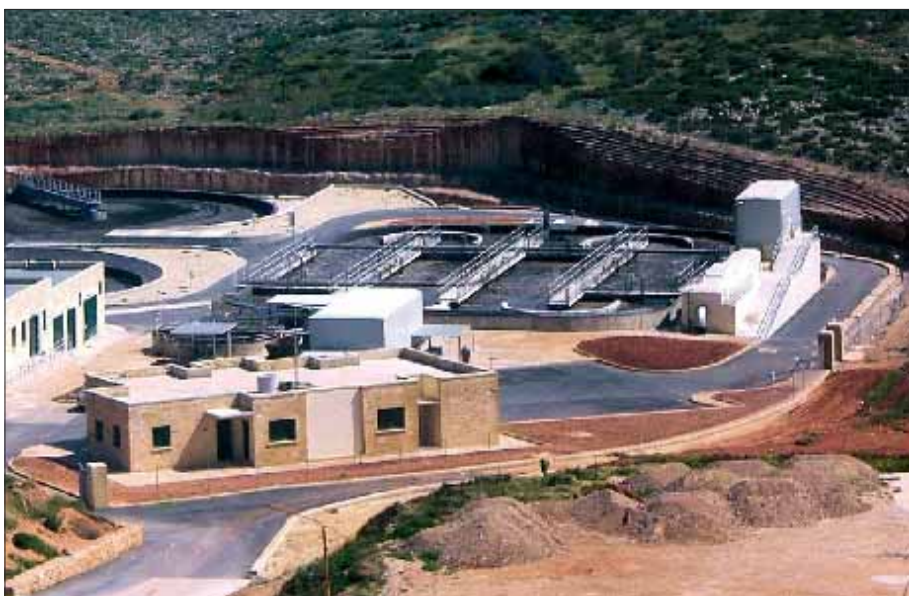
MALTA I.B.I. Waste Water Treatment Plant
